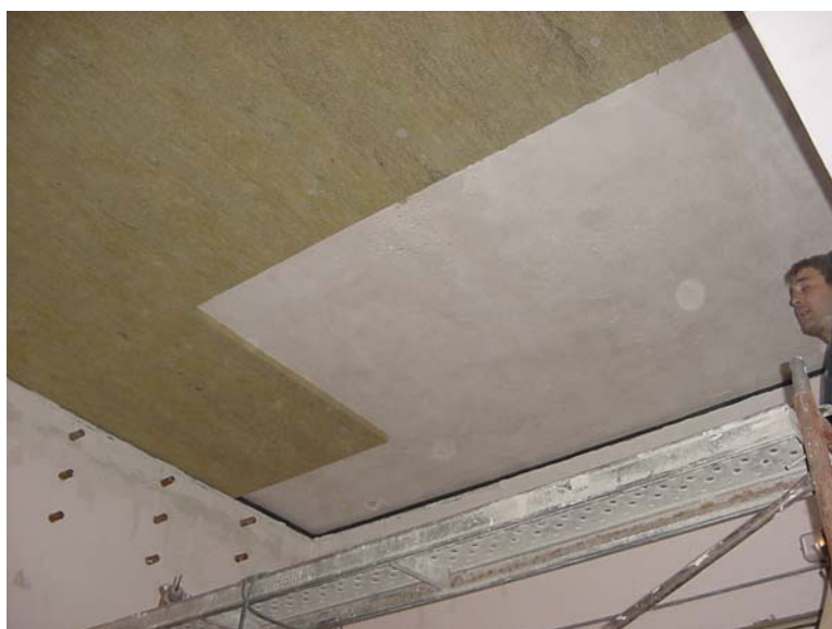
Photo 2: Mounting of the first layer of rock wool
