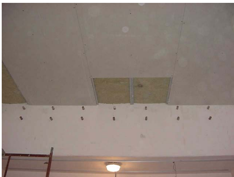
Photo 4: Mounting of plasterboard
