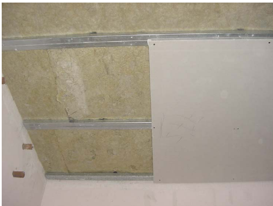
Photo 4: Mounting of the plasterboard
