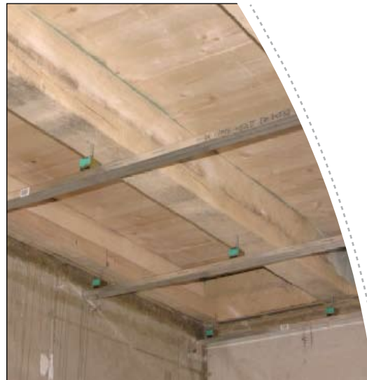
Renovation of wood beam ceilings with Akustik+Sylomer suspension at Laboratory IFT Rosenheim.
