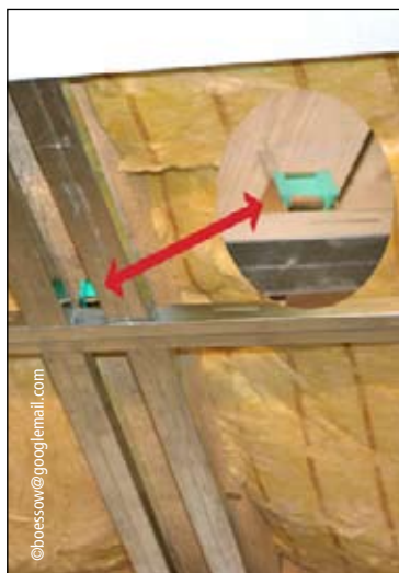
Renovation of wood beam ceilings with Akustik+Sylomer suspension at Laboratory IFT Rosenheim.
